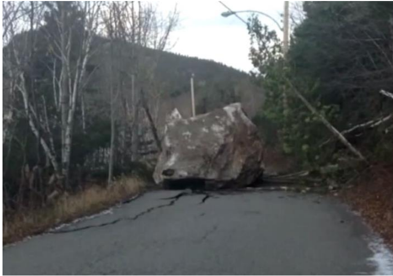
Figure 40. A block, with a volume of 27 \text{ m}^3 , landed on the Chemin de la Mer in Saint-Fabien-sur-Mer, after the 2017 rockfall event (unknown source, TVA Nouvelles, 2017).
