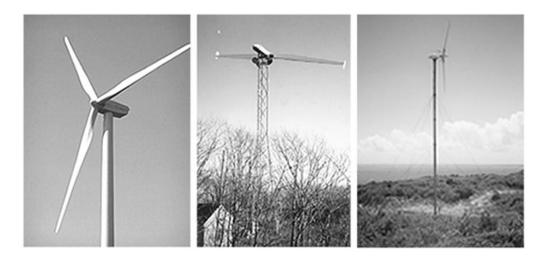
Figure 15. Tubular tower, truss tower, guyed tower (from left to right) [42]
