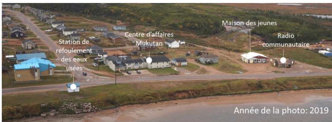
Figure 55: Photo oblique du segment ROM-010, (LDGIZC, 2019)
