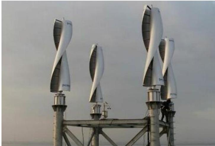
Figure 20. Twisted Savonius turbines
