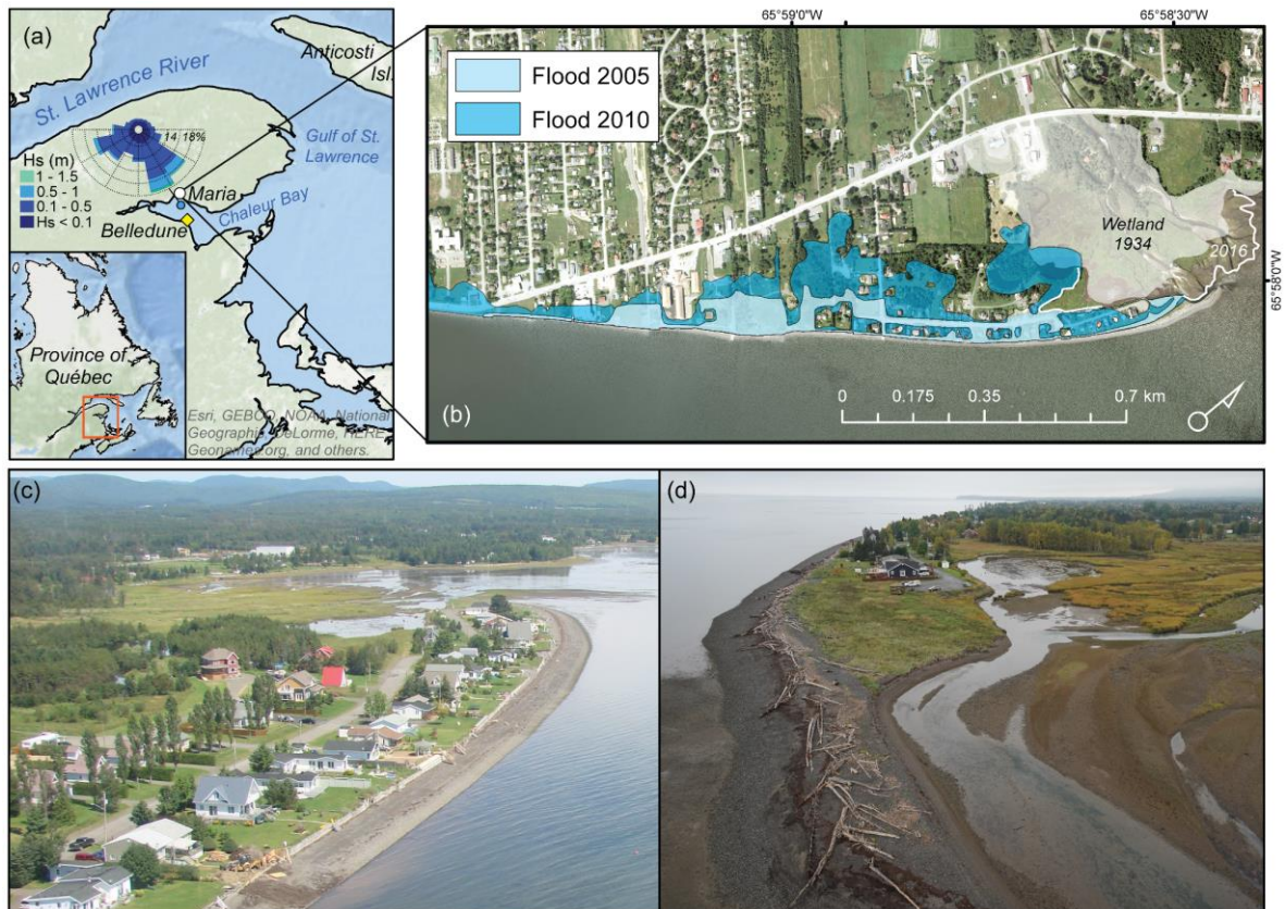
Figure 3.35. Study area location (a) and flooded areas in 2005 and 2010 (b). Airborne photographs (c, d) show the urbanized sandy spit with the wetland. The wave rose is provided by the WW3 hindcast 1983–2010 offshore of Maria (a, blue dot), and the Belledune tide gauge is shown by a yellow diamond.
